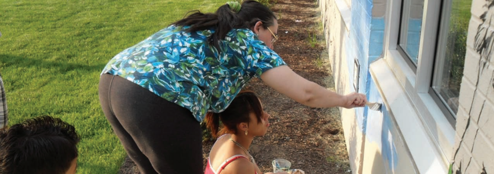
Above: Artist Rosemary Geseck of Bethlehem works with young artists to create a mural on the wall of the newly renovated Cumberland Gardens Community Center.
